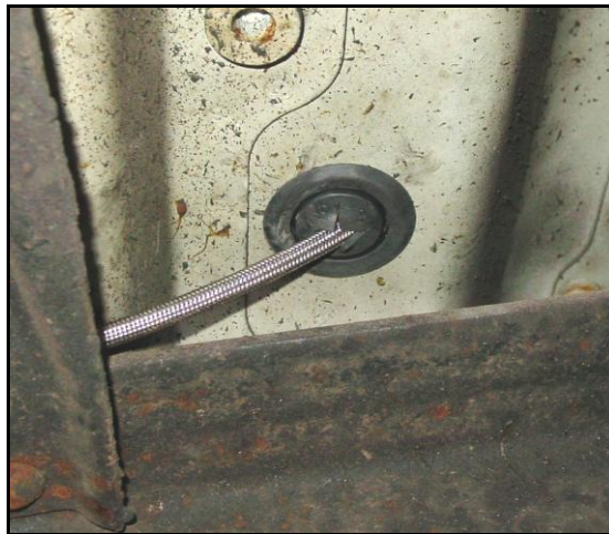
Figure 12 Floor access hole
